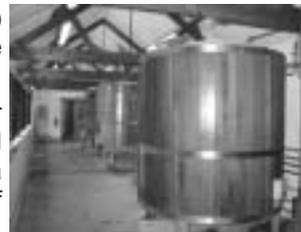
the worts. The beers are fermented in four 400 gallon vessels and five 800 gallon vessels. Three conditioning tanks hold up to 1500 gallons. An old storage barn has been re-thatched and renovated with new beams fabricated from old ships' timbers.
